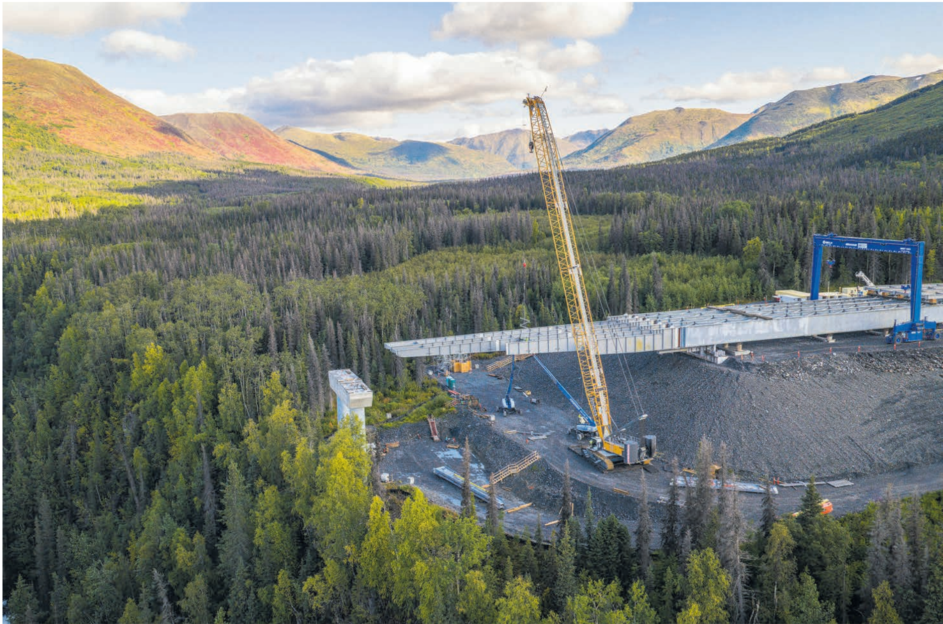
JUNEAU-CREEK-BRÜCKE IN ALASKA
